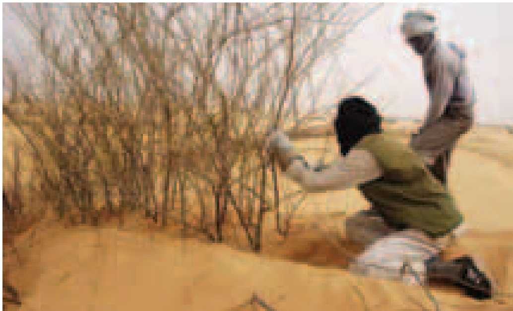
Installing a palisade or fence
